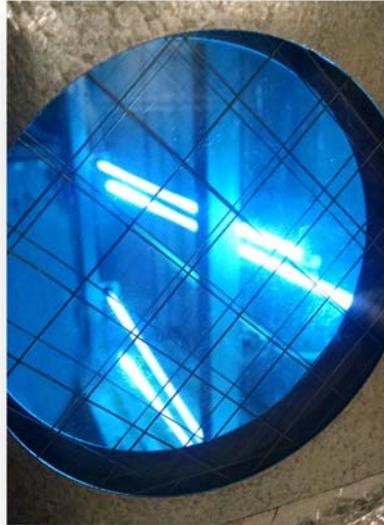
A properly sized and installed set of lamps will noticeably clean a coil in about 30 days with continued improvements up to one year later on severely clogged coils. The UV-C fixtures can be installed in about two hours at an installed cost (materials and labor) of roughly \$0.15 or less per CFM of airflow capacity. For the Kentucky Medical Center, the UV-C installation represented about 10 percent of the cost of a new, replacement coil.
