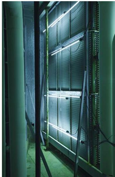
*Similar to fluorescent lamps, modern UV-C lamps use an electric discharge through argon gas that strikes mercury vapor to generate a photon with a wavelength of 253.7 nm.*
